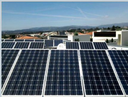
Photovoltaic Solar Energy, Braga, Portugal
