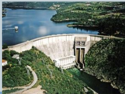
Water Energy, Castelo de Bode, Portugal
